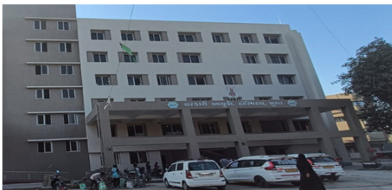
50 bedded Integrated Ayush Hospital, Surat, Gujarat
