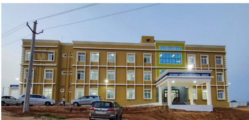
Construction of 50 bedded Integrated Ayush Hospital, Siddhipet, Telangana
