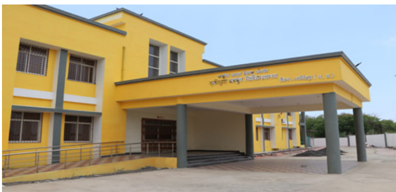
50 bedded Integrated Ayush Hospital at Narsinghpur, Madhya Pradesh
